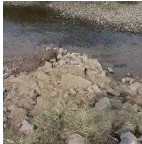
An installed rock groyne.
