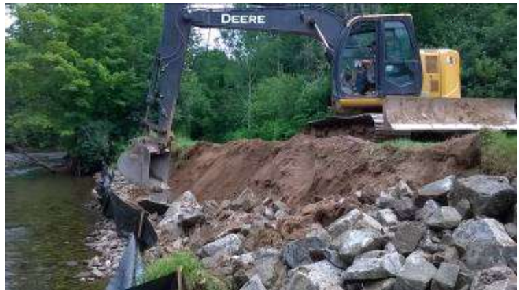
During the summer of 2015, rock was placed by an excavator.
