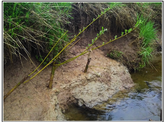
Willow stakes were driven into this degrading stream bank and are now putting up shoots indicating they are rooting into the soil.
