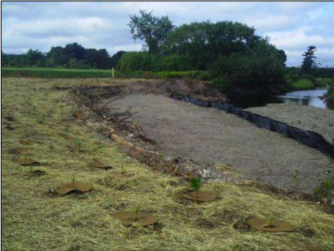
Figure 10: This shows a completed installation of tree revetments. At this location the Millstream River had blown out and caused issues for a crop farmer.
