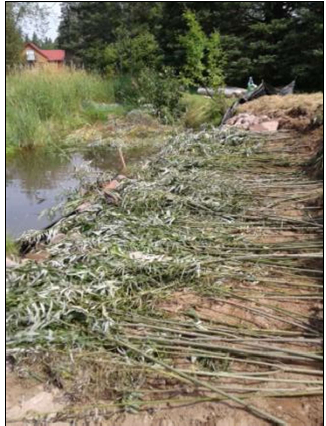
Figure 6: Note the position of the willow stock and the manner in which the bank is prepared.
