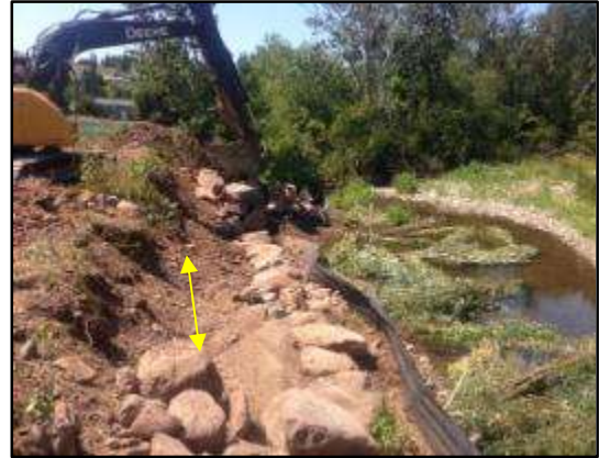
Installing Rock – Rock Groynes are also featured along US & DS portions of this installation.
